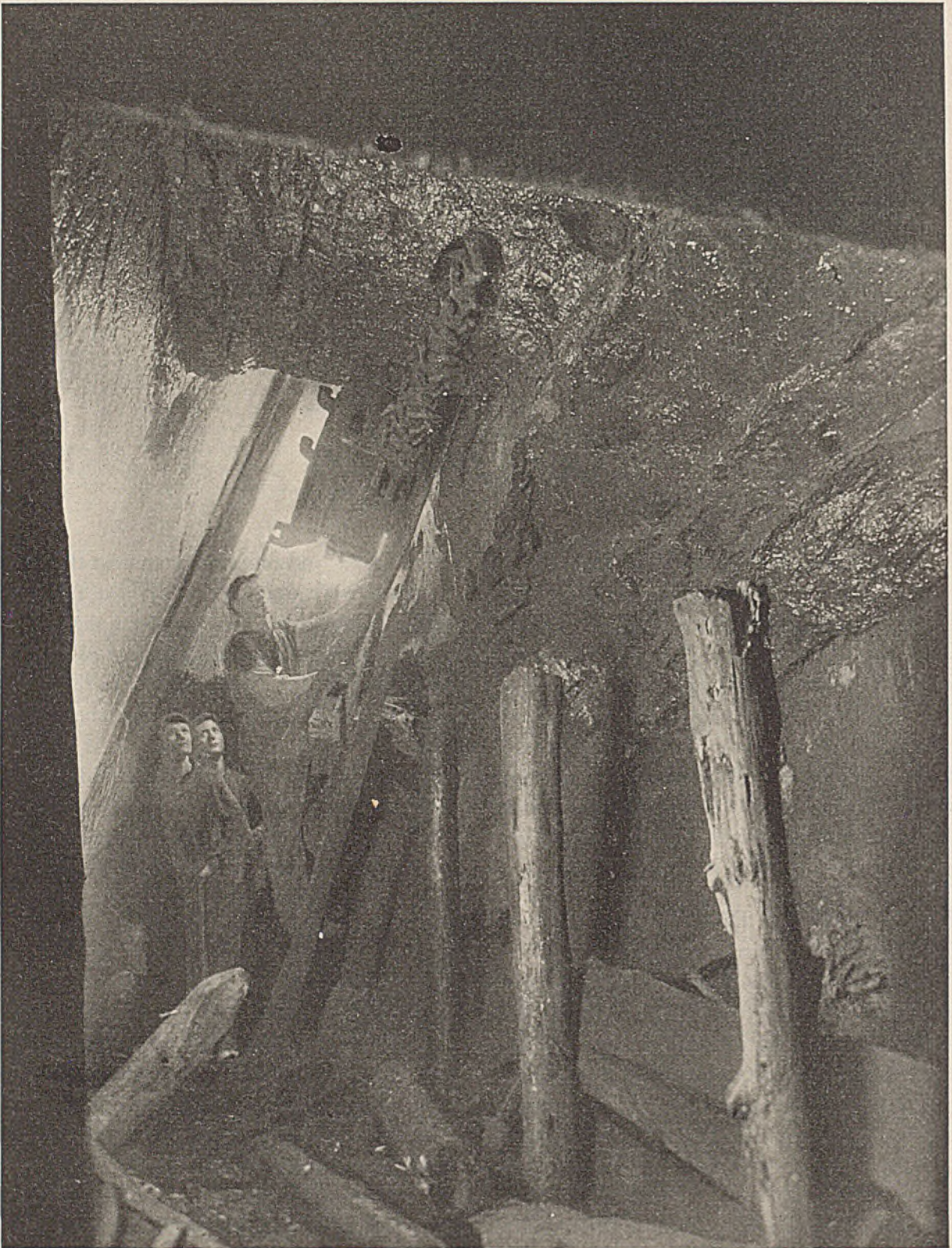
Undercutting a German Coal Bed Which Pitches At Seventy Degrees
