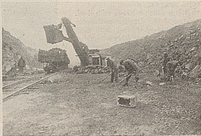
Fig. 2—All Dirt Is Cleaned Off Ahead of the Loader
