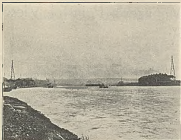
Fig. 12.—66,000 volt Transmission Line: River Tyne Crossing.
