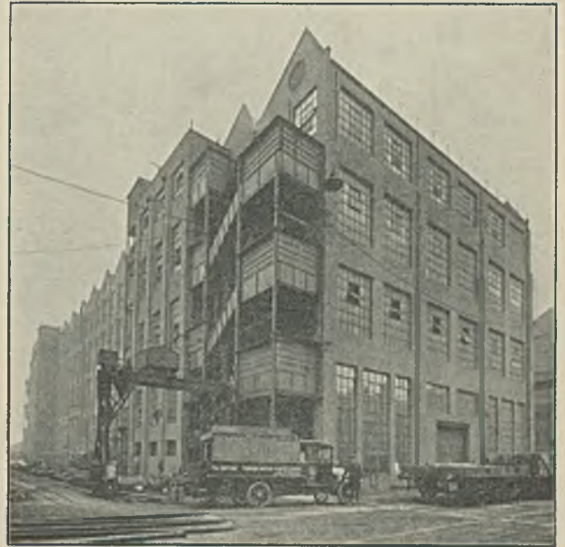
Fig. 1.—The Control Gear Factory.
