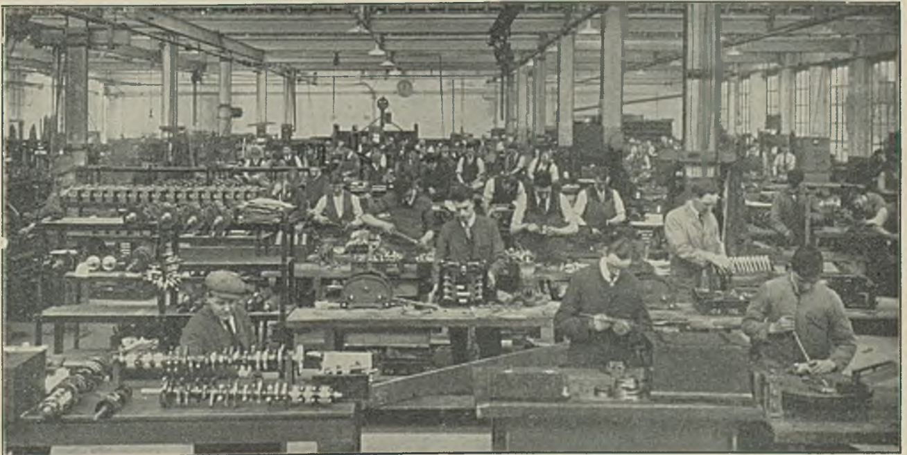
Fig. 2.—Assembling Controllers, Hand-operated Starters, Pillar Starters; also Winding Resistance Tubes.
