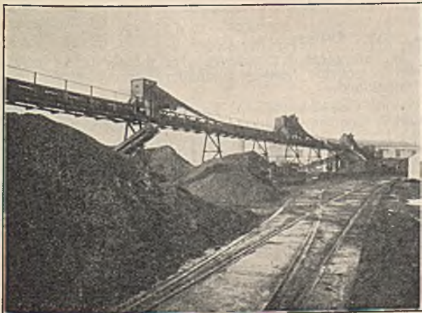
Coal Conveyor: John Westcott, Ltd., Plymouth.
