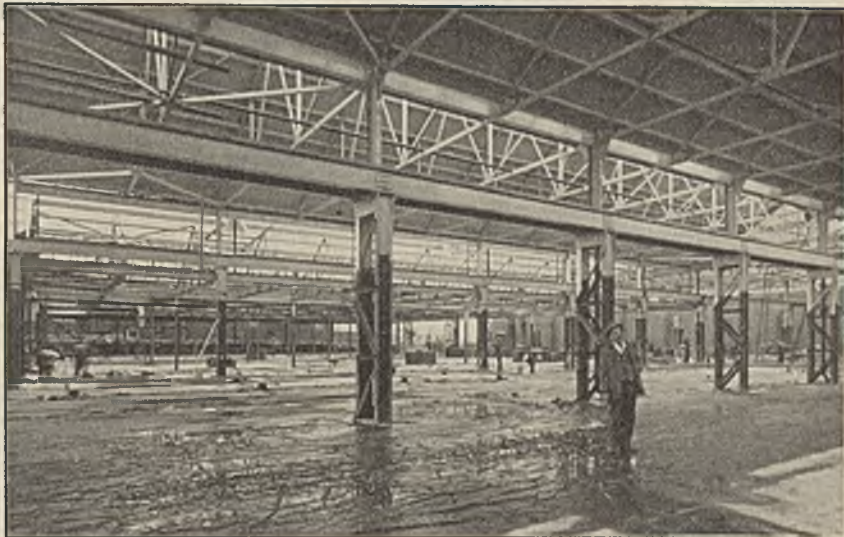
Holmes' Works under construction.
