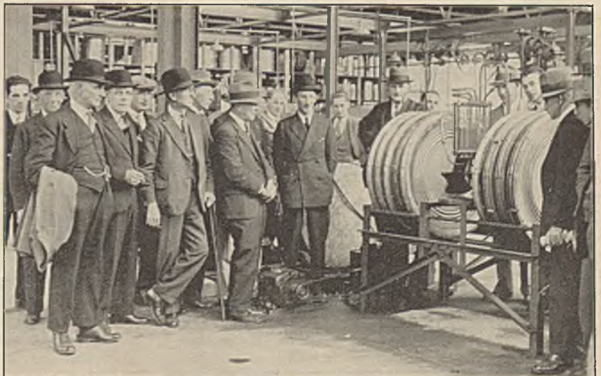
Fig. 5.—Testing Feeding Tank Cells under Vacuum.
