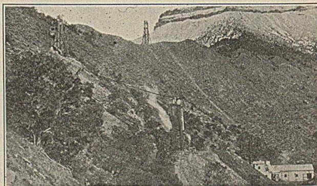
Figure 3—General View of Plant Tramway and Mine Site Mine is on first escarpment in upper right center
