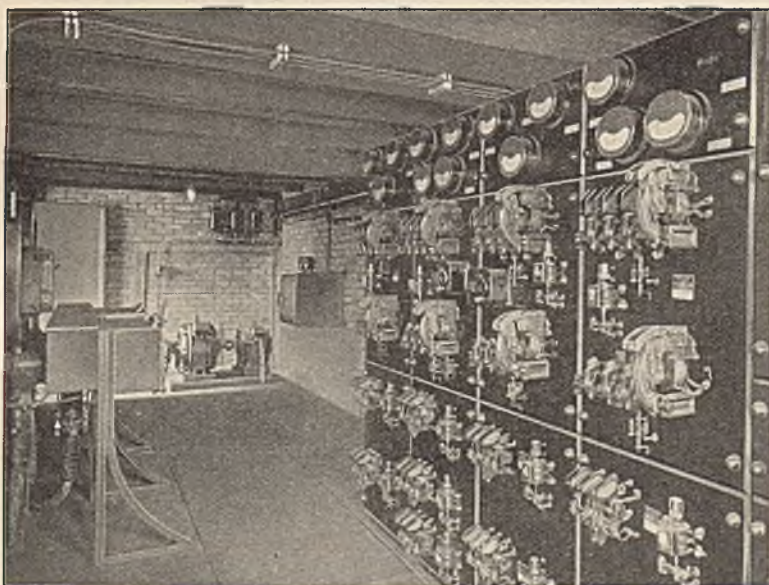
Fig. 21.—Automatic Control for Coal Cleaning Plant.
