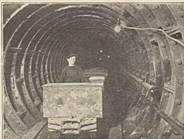
Fig. 6.—Spur-gear drive Locomotive at work in the Hammersmith Sewer.
