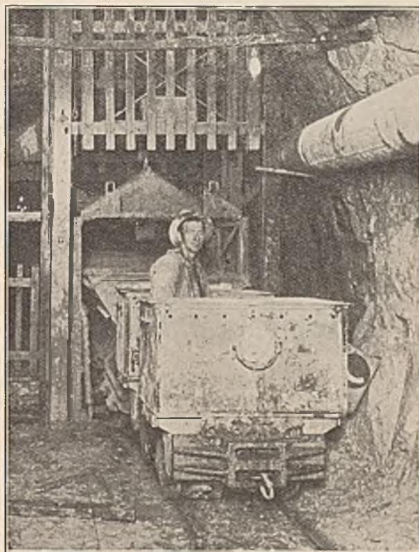
Fig. 1.—Locomotive placing loaded skips in the cage. Sydney Metropolitan Board.
