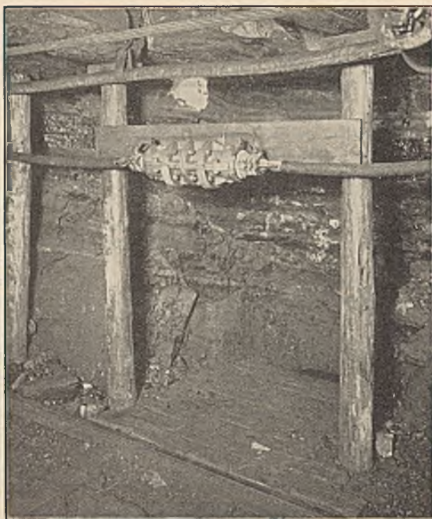
Fig. 1.—Cable Joint made by utilising detachable dividing boxes (Reyrolle).
