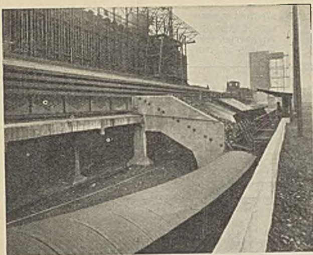
Fig. 7.—A view of the Coke Ovens and Coke Wharf, shewing point of delivery to belt conveyor.
