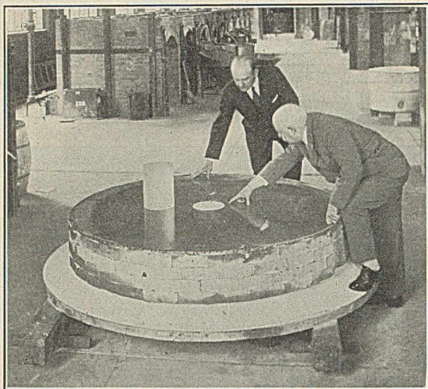
Figure 7—G. K. Burgess, Director of the Bureau of Standards (Right), and C. C. Crump, Professor of Astronomy at Ohio Wesleyan University, Examining the Disk after the Hole Had Been Cut. The "Core" Is Resting on the Surface of the Disk
