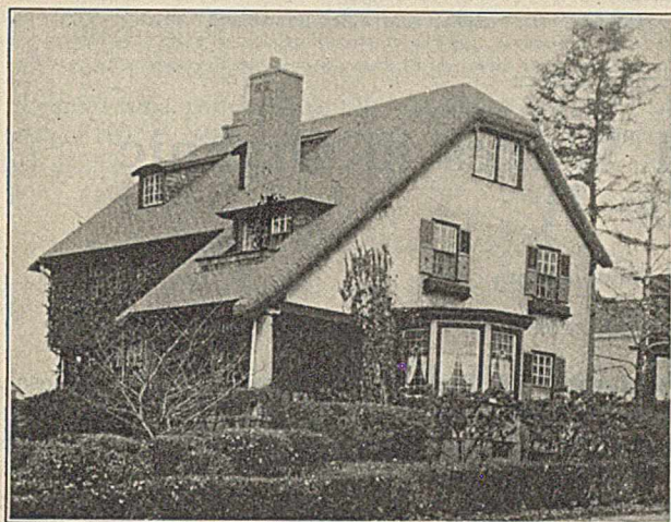
Figure 1—Roof Covered with Multiple Asphalt Shingles
