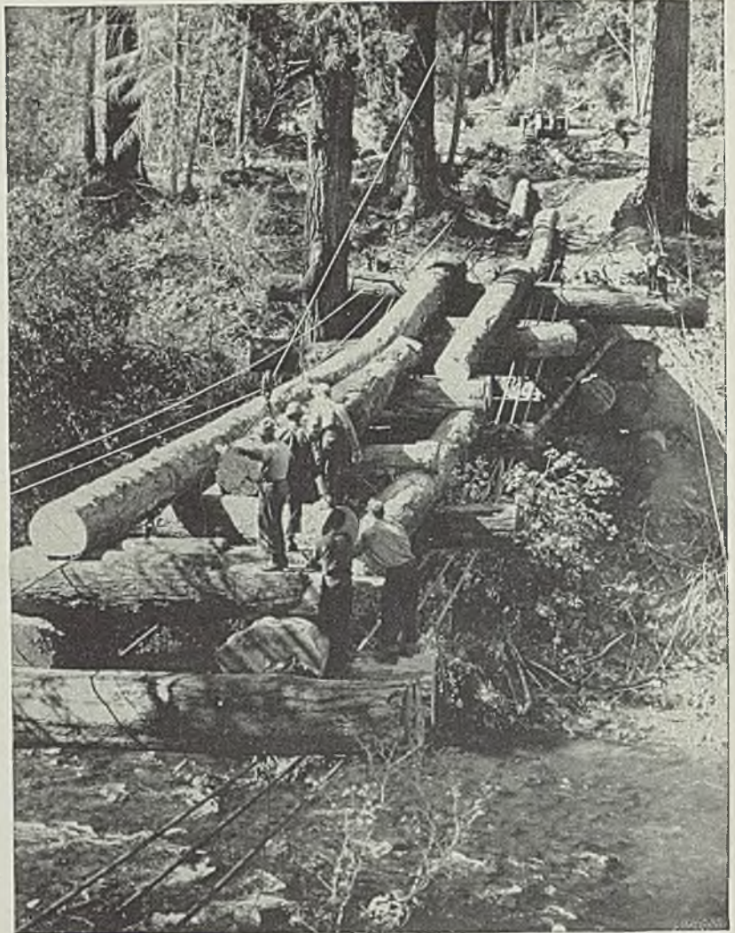
Steel cable plays an important part in modern logging operations. This photograph, taken in Oregon, shows the use of a tractor donkey in the building of a suspension bridge.
