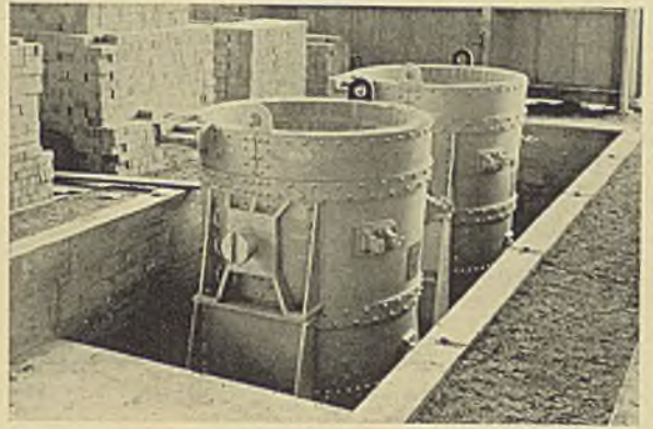
Steel ladles are relined in a concrete pit built near the entrance of the melt shop. Capacity is had for two ladles
