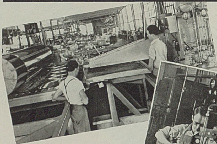
(Top)—At the Boeing Aircraft Co., Seattle, Washington, a Federal Spot Welder is used for making long sheets of aluminum alloy by "stitching" smaller sheets together. Finished work is shown on the roll at the left.
