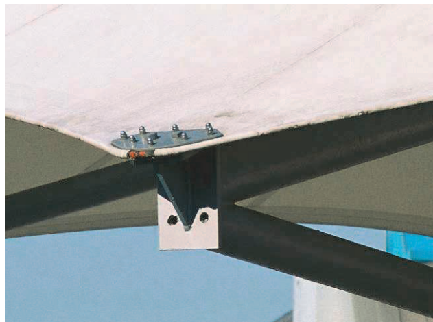
Fig. 6. Fastening the membrane to the corner metal sheet
