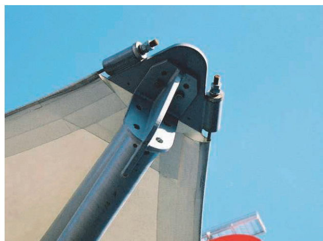
Fig. 7. Adjustable fastening edge struts
