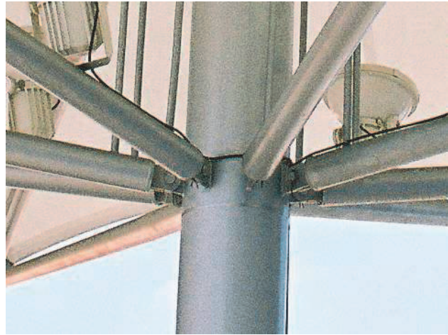
Fig. 5. Fastening of the lower struts
