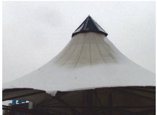
Fig. 11. The small inclination causes snow accumulation
