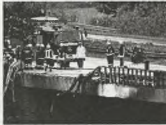
Rys. 3. Uszkodzone elementy balustrad [1] Fig. 3. Destroyed elements of balustrades [1]
