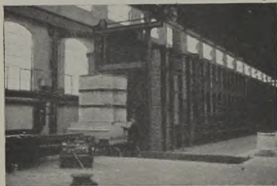
FIG. 14.—TOWN'S GAS FIRED TUNNEL ANNEALING FURNACE.
