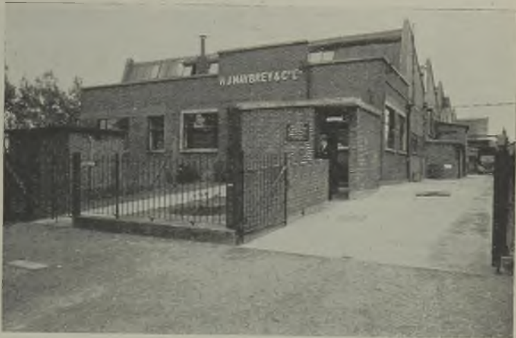
FIG. 1.—FRONT OF OFFICES.
