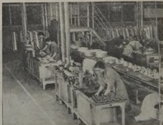
FIG. 50.—GENERAL VIEW OF WATER TEST DEPARTMENT.
