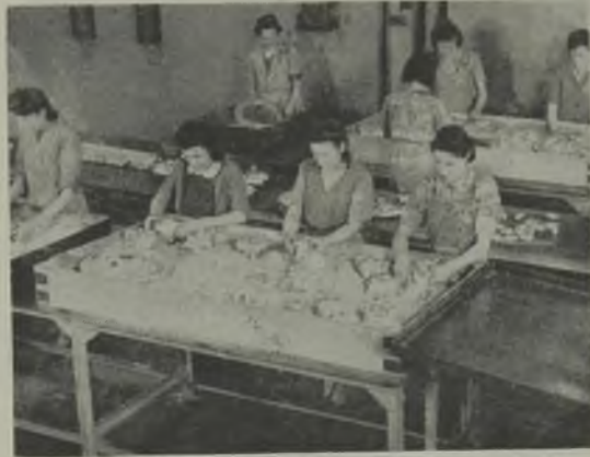
FIG. 40.—CHALK TEST. CASTINGS BEING DRIED AND DUSTED WITH CHALK.
