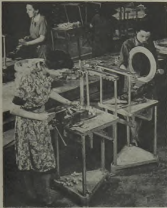
FIG. 47.—TRIMMING OF CASTINGS BY HAND FILE.
