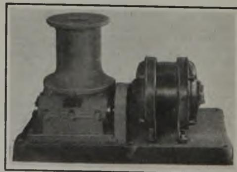
Hoist for Car Placing
