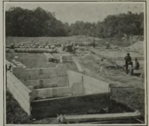
**Fig. 2—Concrete Forms in Storage**
