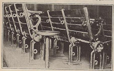
Frames Are Made of Cast Iron and Set in Concrete
