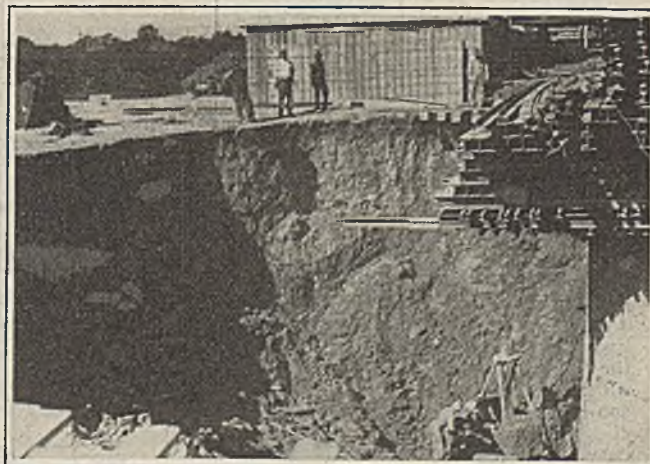
When the Shaft Lining Began to Tip
