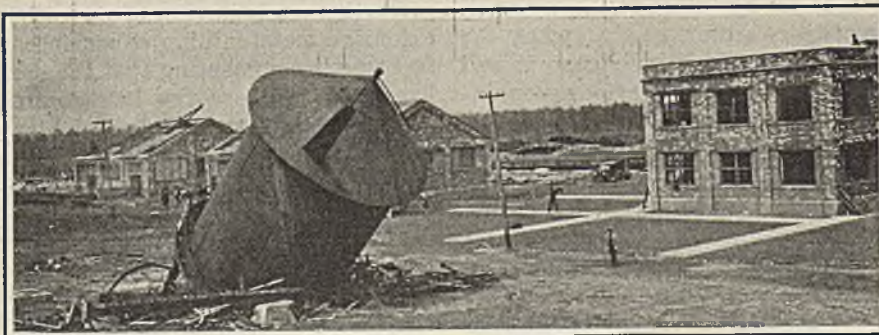
How Water Tank Collapsed at New Orient When Tornado Struck It
