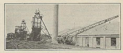
When the Tornado Did the Lifting the Crane Left the Railroad Tracks At New Orient Mine of the Chicago, Wilmington & Franklin Coal Co., after the tornado of March 18. From left to right: Main holst, auxiliary hoist and boiler room. Note how well the steel structures, despite their covering, withstood the tornado. The concrete stack, also, successfully battled with the storm.
