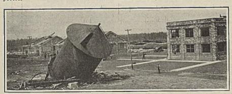
How Water Tank Collapsed at New Orient When Tornado Struck It
