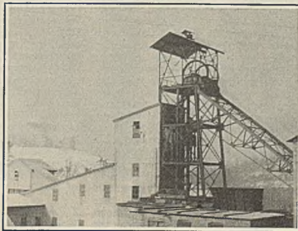
Steel Headframe and Tipple, Cranberry No. 1 Mine
